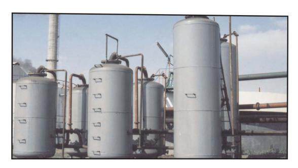
Tertiary system to streams 100 M³/hr. each Power sand filter followed by plant based activated carbon & polishing unit comprising high grade anthracite and activated carbon
