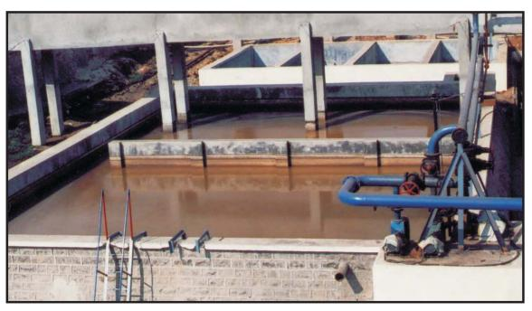
New equalization tank and feeding system to old and new stream 20 M³/hr.+ 70 M³/hr.
