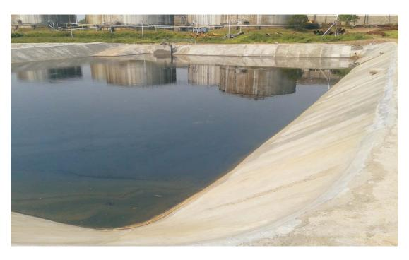
R.C.C. with Geomembrane paper lining laid for Lagoon No.1
