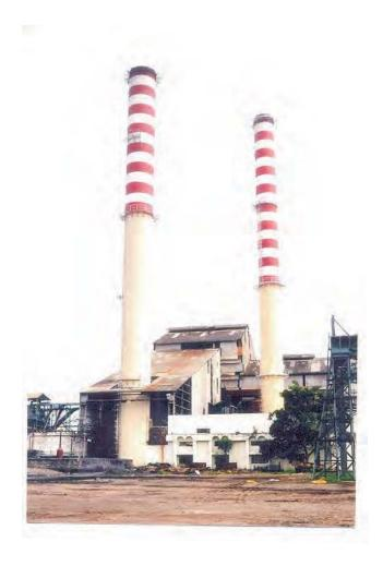
90, 20 & 75 M.T. /hr capacity Boiler Chimney. 75 Mtr. and 72 Mtr. Height respectively
