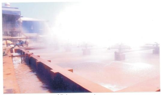
Mini spray pond capacity 10200 M³/day water recycle inlet temprature 58°C to 60°C outlet temprature 28 to 30°C
