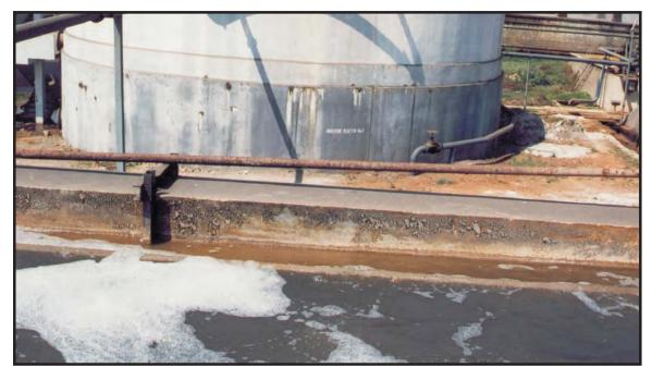
New anaerobic counter current digester 70 M³/hr. and preareation tank outlet
