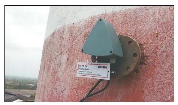
Dust monitor unit for Total Particulate Matter for stack
